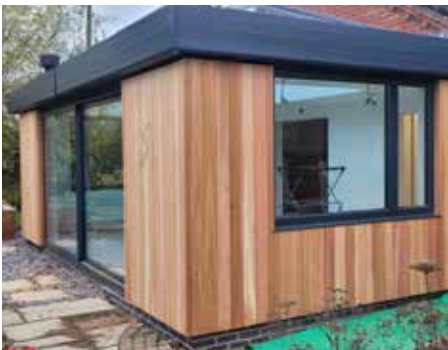
Vertical Timber Boards
