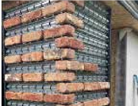
Brick Slips rail application
