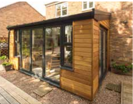
Horizontal Timber Boards
